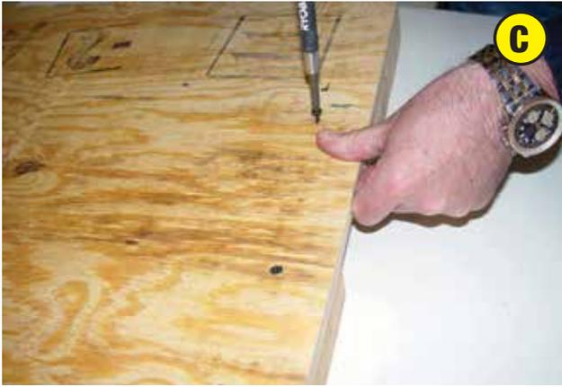
Use 2" screws to secure the 2" x 4" x 10" blocks from the underside.
