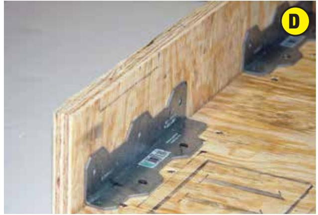
Glue and screw (with 2" screws) the 6" x 24" piece of plywood across the front as shown. Use 2" x 6" (or 8") stair angles for reinforcement. Secure with screws.
