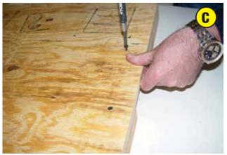
Use 2" screws to secure the 2" x 4" x 10" blocks from the underside.
