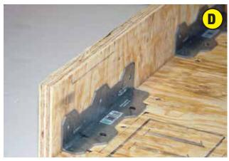
Glue and screw (with 2" screws) the 6" x 24" piece of plywood across the front as shown.
