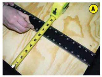
Using a 24" x 24" x ¾" piece of plywood cut a 6" x 24" section of the plywood for the front edge brace.
